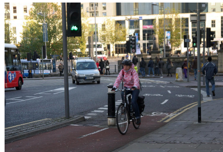
Two Way Cycle Lane Across Light Controlled Junction" by samsaundersbristol is licensed under CC BY-SA 2.0
