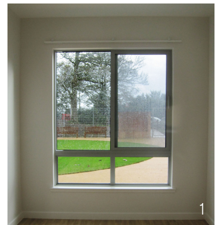
Window with secure sliding panel.
