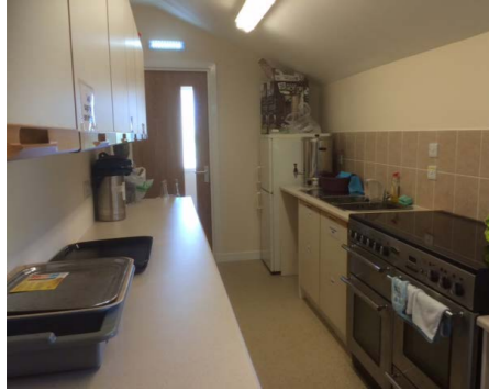
Kitchen after refurbishment
