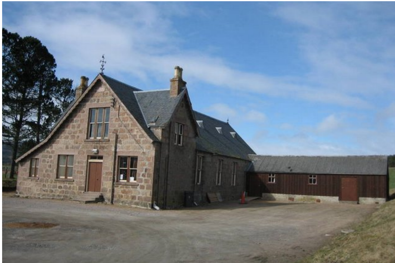
The hall before the work, with later ^ timber small hall.
