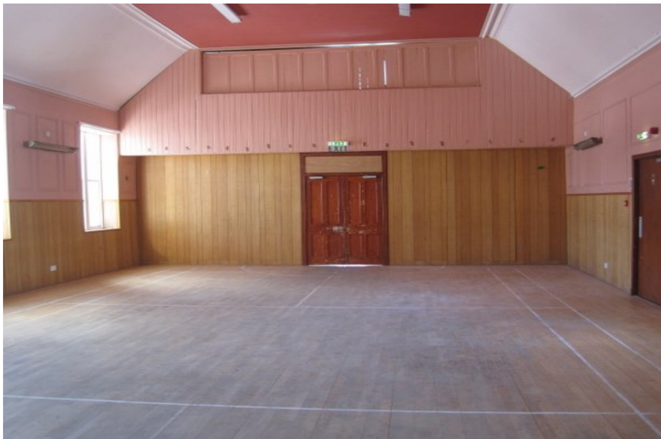
View of main hall before the work v
