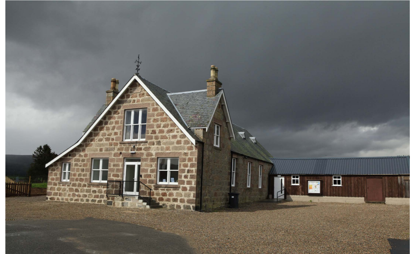
^ External view of refurbished Logie Coldstone Village hall
