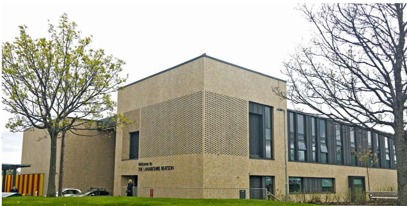
View towards the main entrance from the access road
