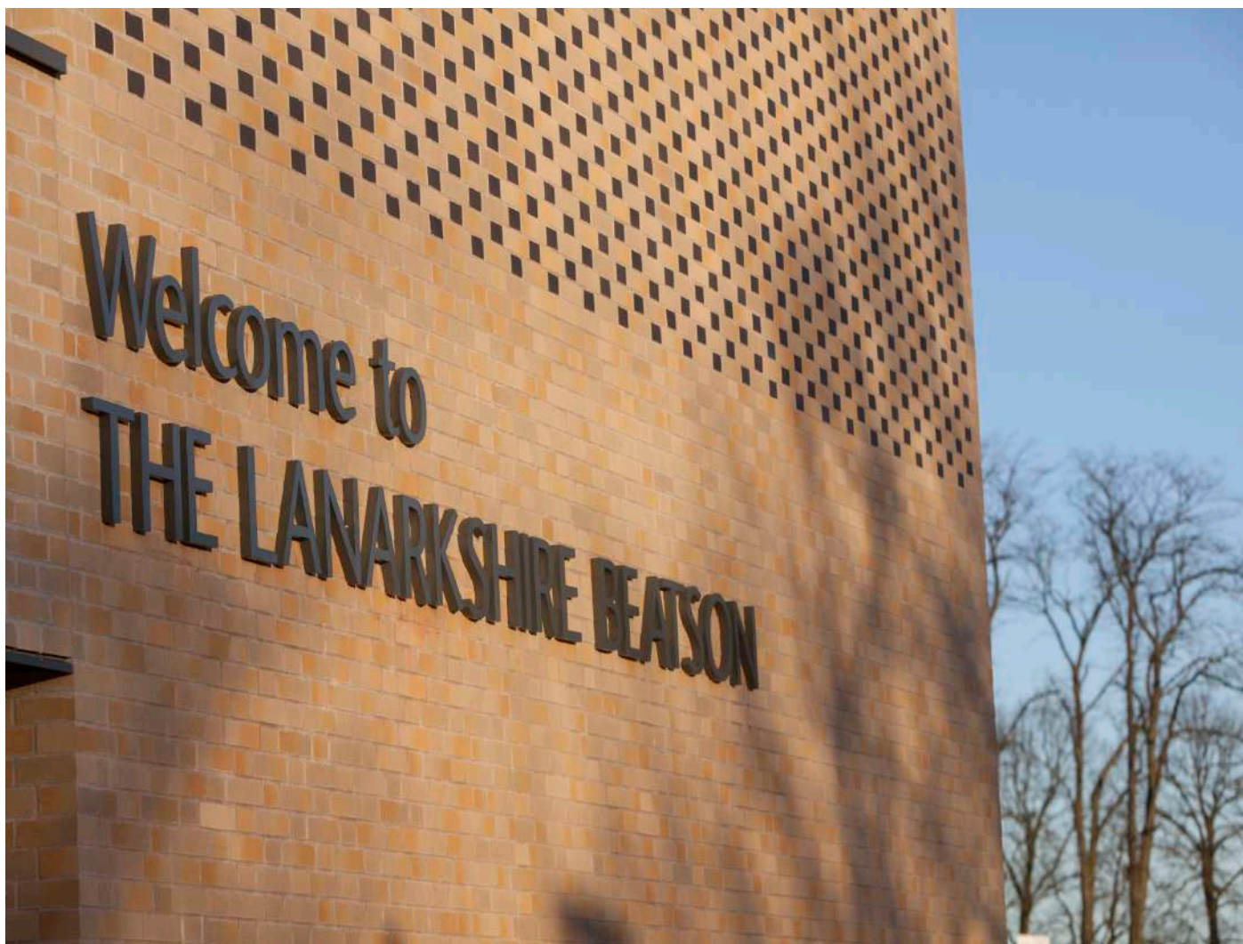
Natural Buff Brick Cladding provides an appealing aesthetic within a tight build schedule
