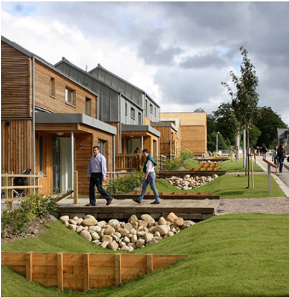
^ Swale integrated into the streetscape.
