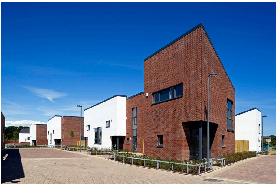
^ Corner marker house
