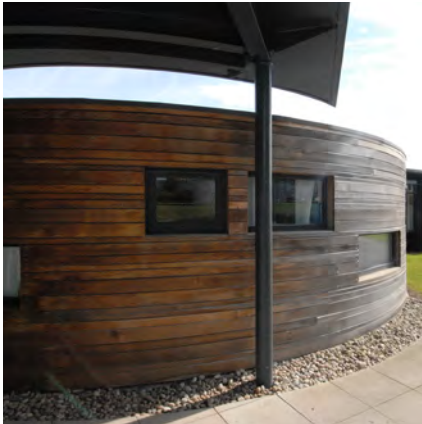
^ The entrance drum at Muirview Image credit: A+DS
